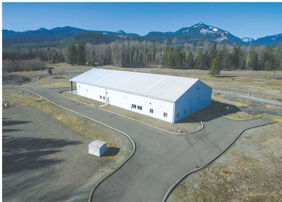
The East Lewis County Public Development Authorities Packwood property is up for lease. A potential award-winning brewpub is taking a serious look at opening at the property.
