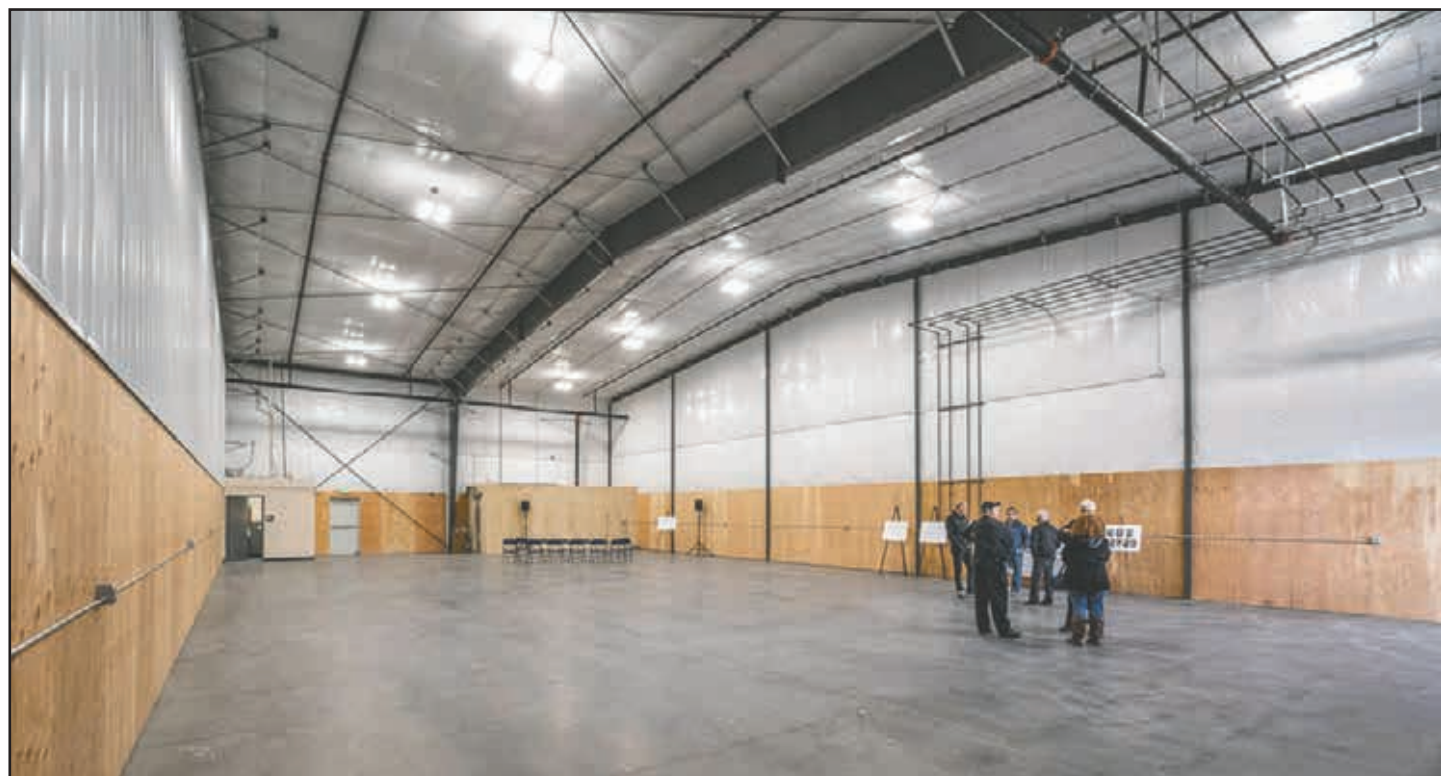
The inside of the Pomerl Building in the Chehalis Industrial Park is pictured in this photograph provided by the Port of Chehalis.
