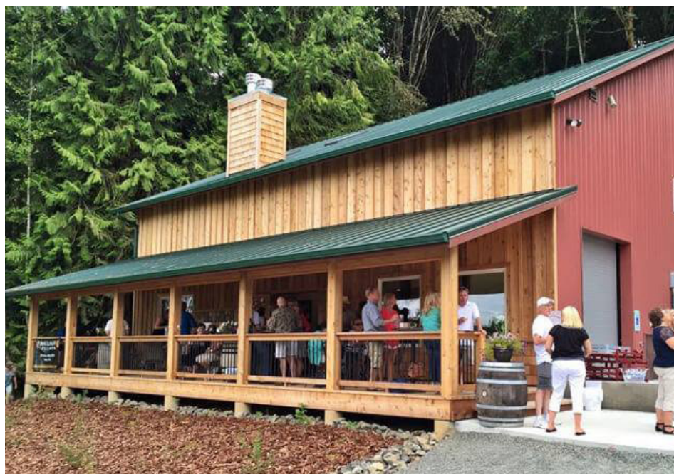
Bateaux Cellars tasting building
