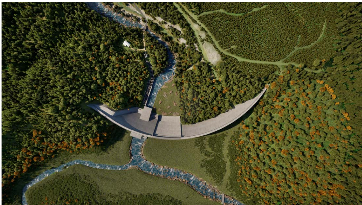
Aerial view of the flood-through dam.
